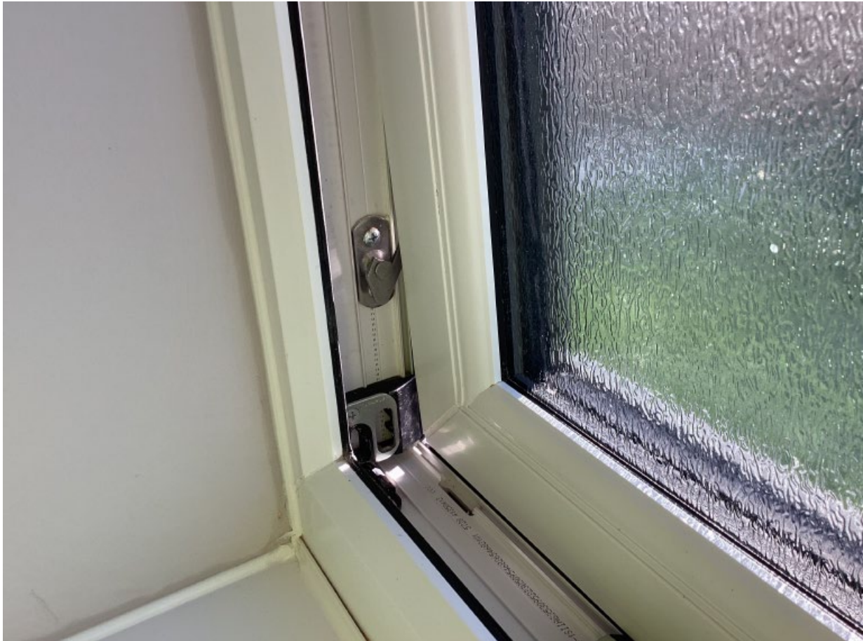
Fig 4: A001 Quick Release Restrictor (example)
