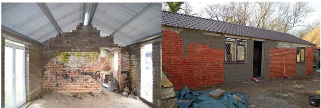
Internal/External photograph showing large areas of elevation built up with new block work, new roof and windows. (photo suppled by applicant)
