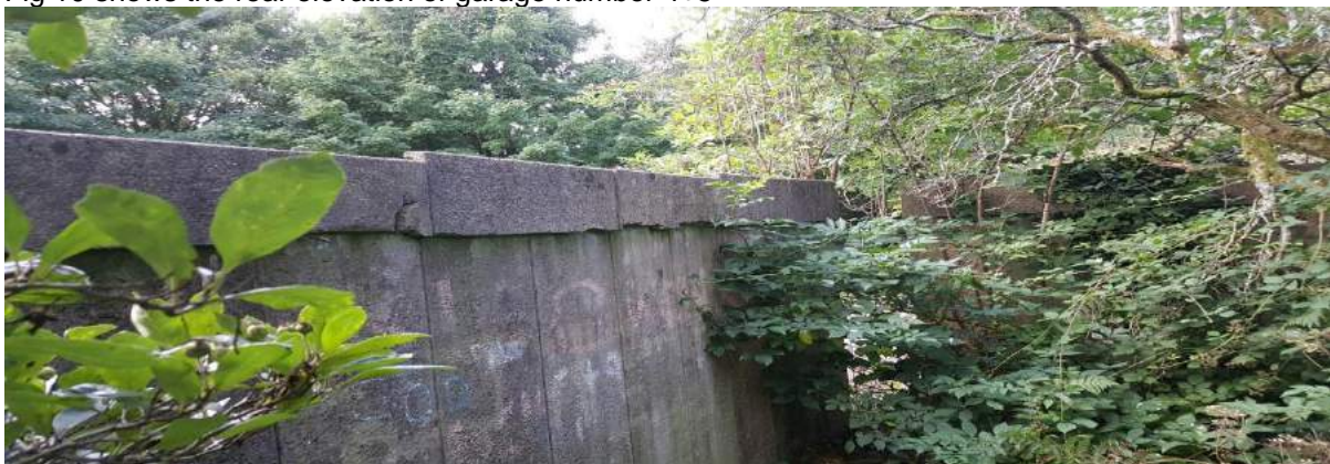
Fig 11 shows the rear elevation of garage number 1-3 with the decayed concrete fascia and overgrown vegetation
