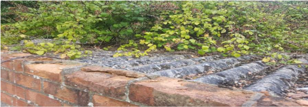
Fig 13 shows the roof of garage 1 and the poor state that it is in along with the splitting of the clay bricks.
