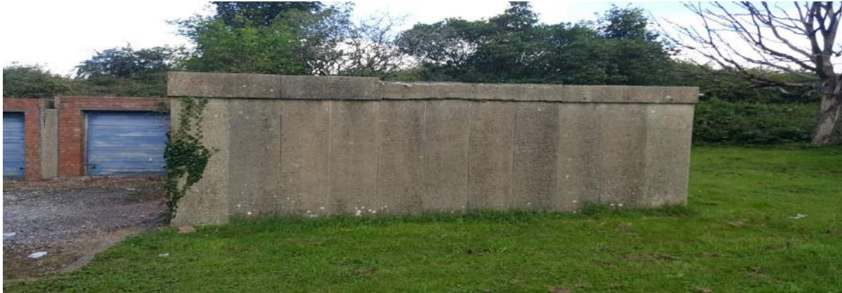
Fig 9 shows the side elevation of garage 5 and the state of the precast concrete panels
