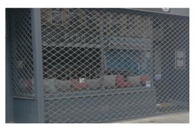
Figure 13: Example of External Lattice Type Shutter
