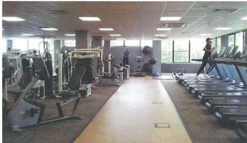
EXISTING VIEW FROM ENTRANCE 1: THE DATED CARPET AND VINYL FLOOR FINISHES ARE TO BE REPLACED WITH CONCRETE-EFFECT VINYL TILES THROUGHOUT
