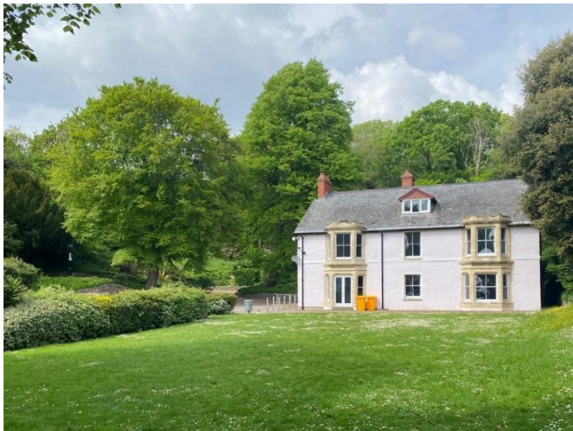
Front (south) elevation of The Kymin
