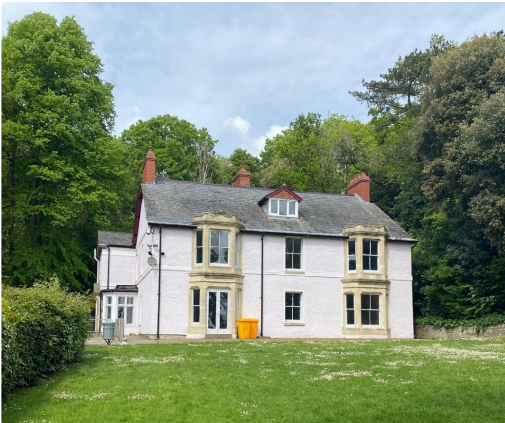
Front (south) elevation of The Kymin.
