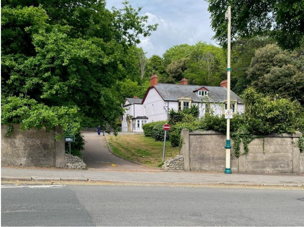
Front (south-west) elevation of The Kymin).
